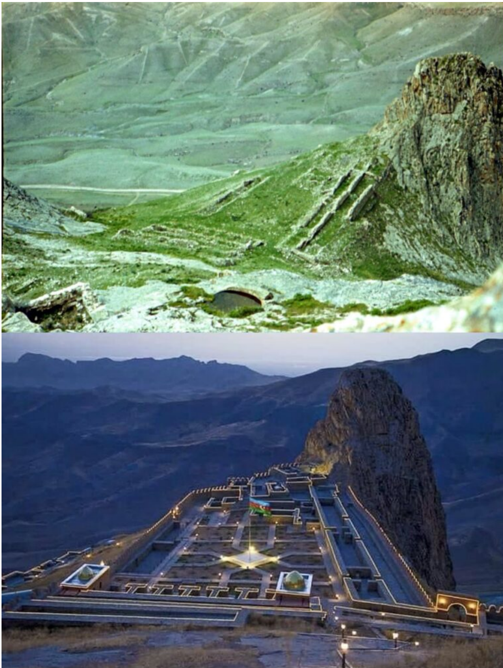
Foundations of the 7th century Yernjak (Θlinca) fortress in 1970s and its 'brand new' look today. Courtesy Argam Ayvazyan.
